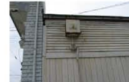
21. Missing downspout, rusted gutter and peeling paint. Replace downspout and gutter, scrape and repaint.
