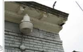
16. Metal gutter deteriorating and wrong lighting. Replace gutter and install appropriate lighting.
