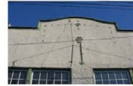
Cracks in stucco, off-center signage support, dissimilar stucco. Repair cracks and resurface stucco, remove sign support.
