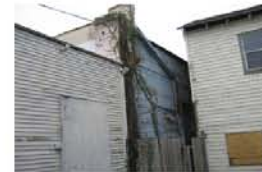
6. Broken gutter system and evasive vegetation, rotted siding. Install new gutter system, remove vegetation, metal siding and repair chip-board siding.
