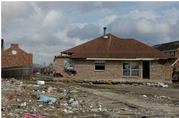
Figs. II.D.16–18 Slab on grade houses damages or washed away by flooding
