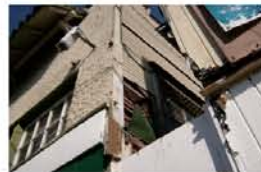
Metal siding, damaged clapboard, and rotting trim boards. Remove metal siding, repair and paint clapboard and trim.
