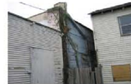
Evasive plant life, deteriorating gutter system, metal siding. Remove vegetation, metal siding and replace gutter system.
