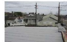
14. Damaged flashing roof recently replaced. Inspect and replace damaged flashing.
