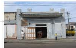
13. Storage room windows covered and wood trim rotting. Replace rotting wood and uncover windows.
