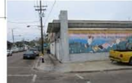
22. Windows covered, gutter rusting, evasive plant growth. Remove and save mural, repair gutter and remove vegetation.
