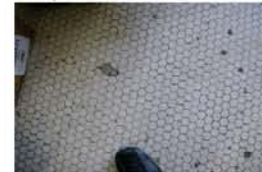
9. Missing broken tile and water stains. Replace tile and clean, disinfect and seal floor.
