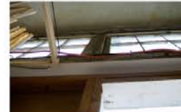
2. Structural damage and window degradation. Consult with engineer for solution to structure damage, repair window.
