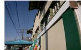
3. Showing bow of front facade and condition of stucco. Consult with engineer for bow, repair stucco and wood.
