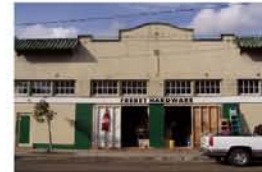
8. Temporary plywood doors, chipped eyebrow tiles. Replace with operable door and replace tile.
