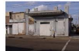
17. Plywood door, transom and window covered. Replace door, uncover transom and windows.
