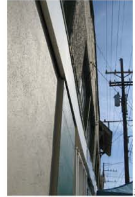
Bow of front facade. Consult with structural engineer for reasonable solutions.
