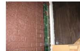
15. Painted brick and missing tile and window covered. Replace missing tile, open windows remove paint from tile.
