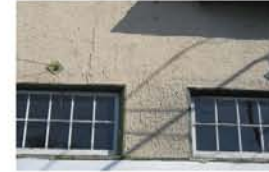
Cracks in stucco and multiple textures, rotting trim. Repair and resurface stucco, replace rotting trim.
