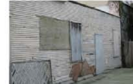
23. Window covered, rotting wood, paint peeling. Repair windows, replace siding and repaint.
