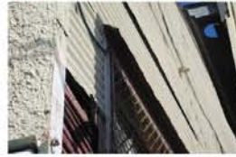
Original/Temporary siding, chain link fence over windows. Remove metal siding, restore wood clapboard, remove fencing.
