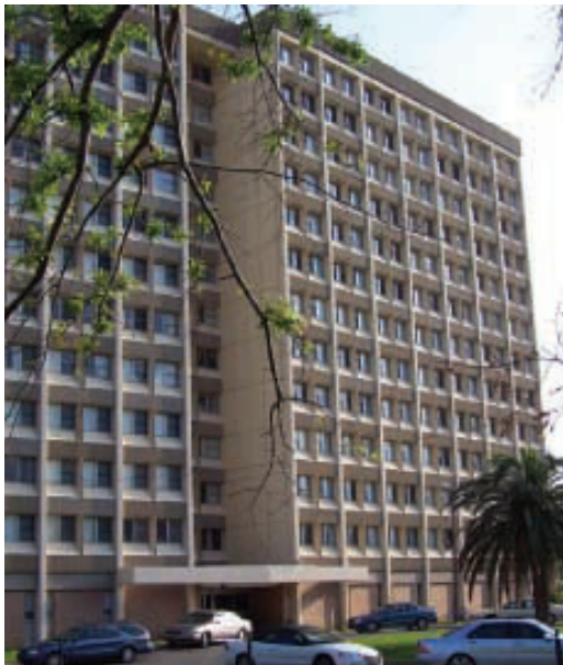
Reinforced concrete building that performed well under wind loads (lower left); wooden frame residential structured damaged by winds (center and right images)
