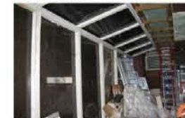
18. Store front glass covered, missing ceiling tile. Uncover glass and replace missing ceiling tile.
