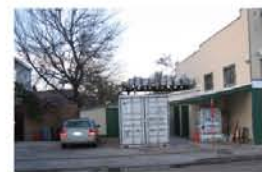
5. Temporary storage unit, water damage at corner of building. Remove storage unit, manage inventory, repair corner of building.
