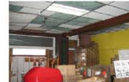
20. Missing ceiling tiles, water damage to ceiling. Repair water leaks and replace ceiling tiles.
