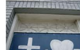
24. Painted windows and trim. Remove paint from windows and repaint trim.
