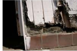
Rotted wood siding and paint on tile. Replace siding and damaged framing, clean tiles.
