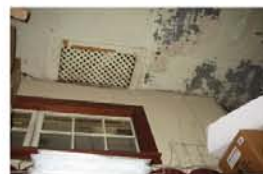
WATER DAMAGE
