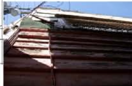
10. Peeling paint and rotted wood. Replace rotted wood, scrape and paint.
