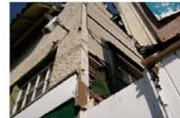
11. Wood rot and stucco damage. Replace rotted wood and patch stucco.
