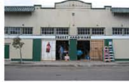
Temporary plywood doors. Replace with operable door system.
