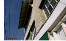
Spanish tile eyebrows, missing awning, wood damage. Repair tile eyebrows, replace awning and wood window trim.
